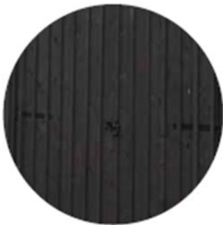
PAINTED TIMBER CLADDING
