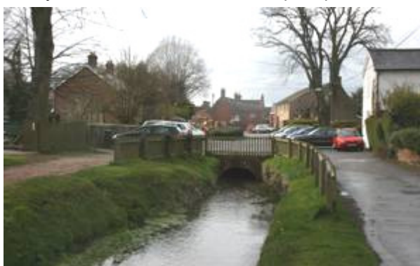
Figure 19: View of the River Crane emerging from its culvert beneath Crane Street .
