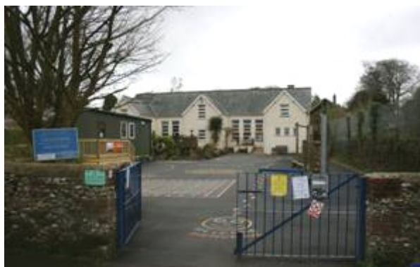
Figure 20: View of Cranborne CE VA First School, Water Street.
