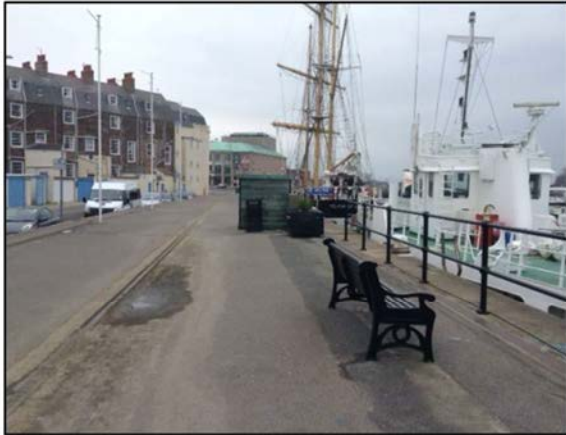
Commercial Road (south)
