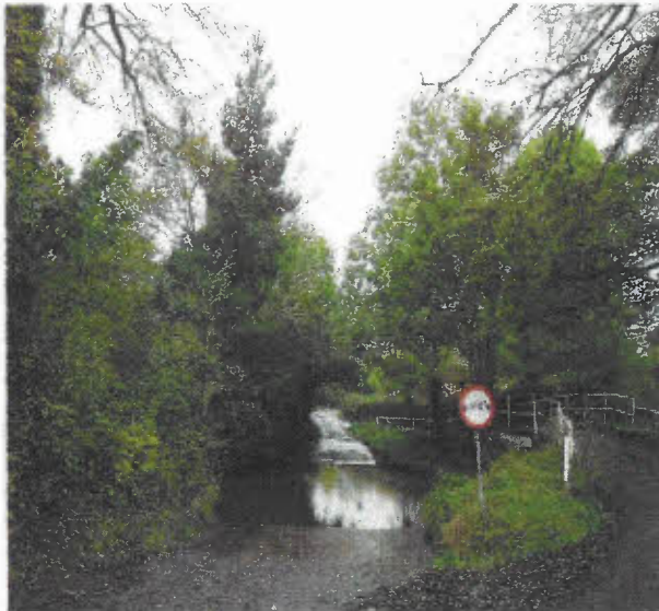
Photo 36 – Colesbrook Lane – 'ford' – east approach
