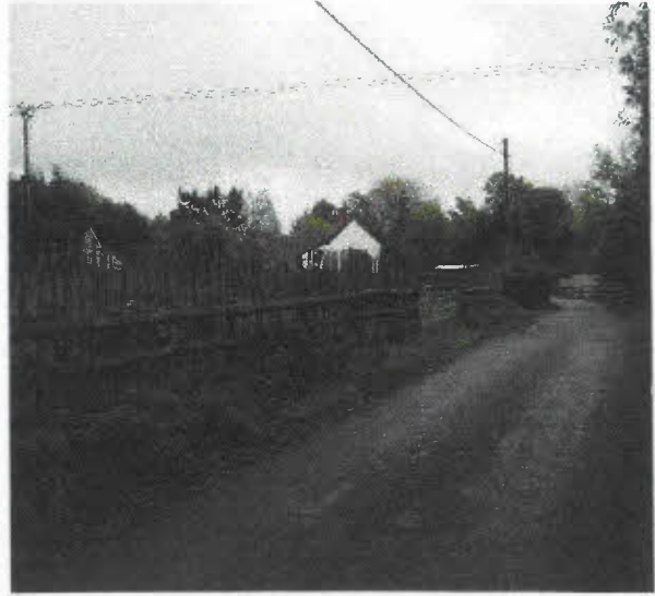
Photo 32 – Colesbrook Lane – abandoned plot on left stripped of any trees and other vegetation.
