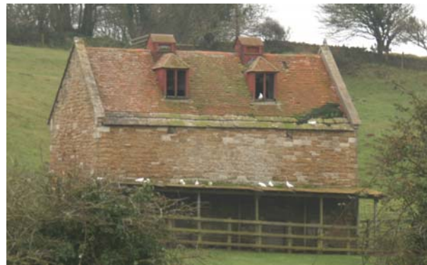
Figure 49: The Dovecote, Abbey Farm.
