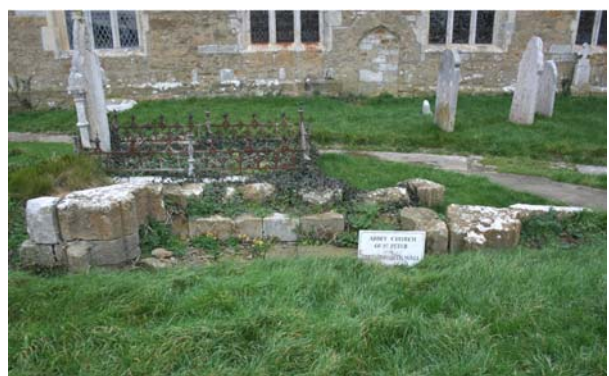
Figure 16: The exposed part of the north aisle north wall of St Peter's Abbey church.
