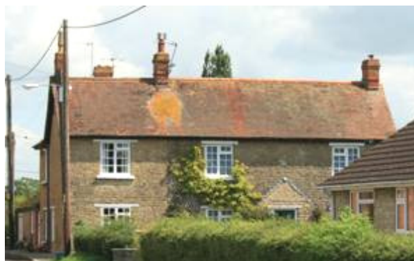
Figure 66: Kings Cottage, Kingscourt Road.
