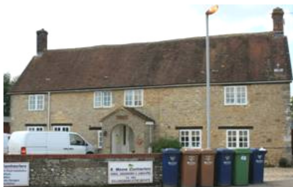
Figure 64: Higher Ham Farm House, Shaftesbury Road.
