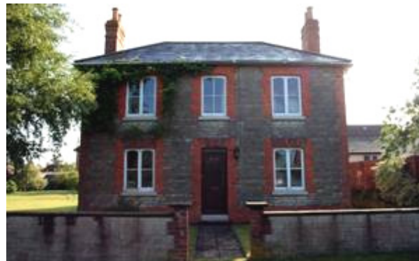
Figure 80: Tresillian, Bay Lane.
