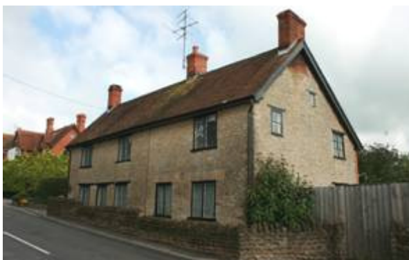
Figure 95: Old Toll House, Wyke Road.
