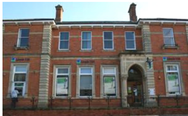
Figure 50: Lloyds Bank, High Street, Newbury.
