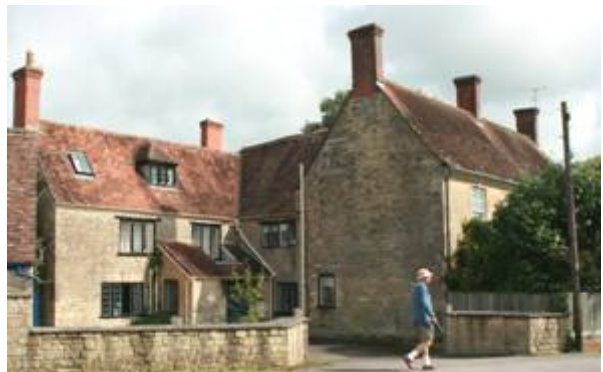
Figure 43: Plank House (right) and River Gate (left), Wyke Road.
