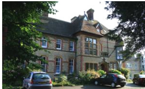
Figure 42: View of the Vicarage (Rawson Court), Queen Street.
