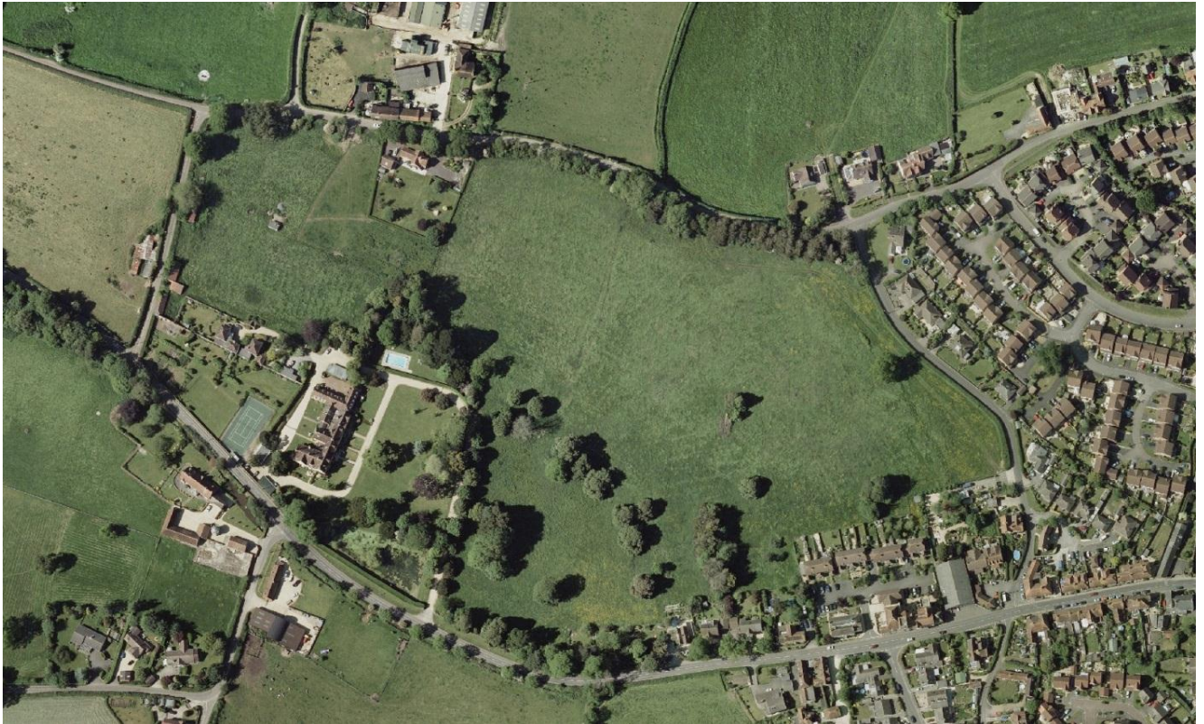
Aerial view of Wyke Hall and its existing and former grounds. The curved row of trees within the centre of the photograph indicates the position of the former access to the Hall. Slaughtergate Farm lies to the north.
