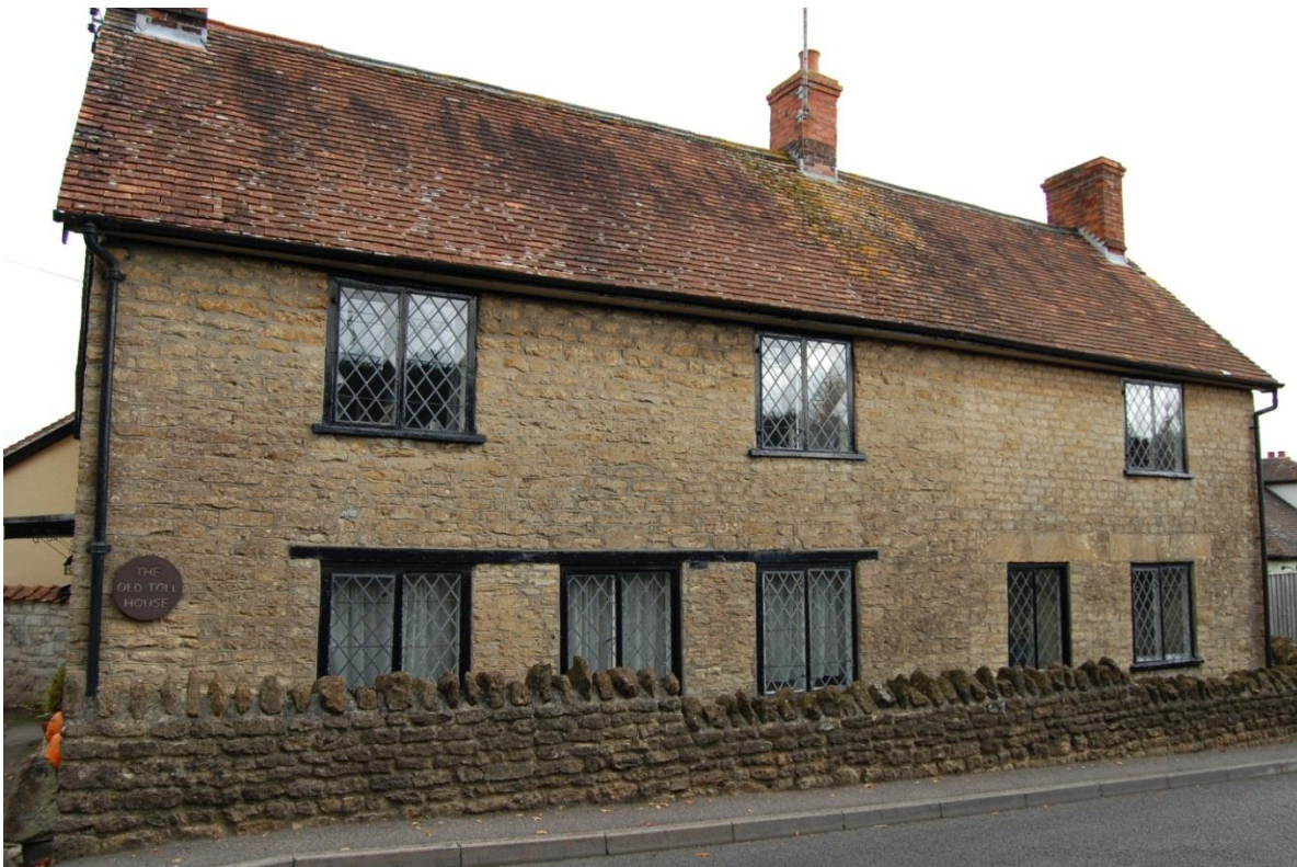
The Old Toll house, an example of the local vernacular located at the eastern end of the conservation area. The windows have been altered and the property extended but it is still a valuable heritage asset.
