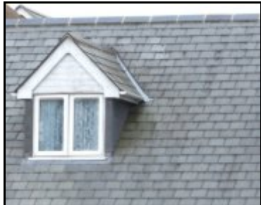
37 Recent slate roof at Breach Close
