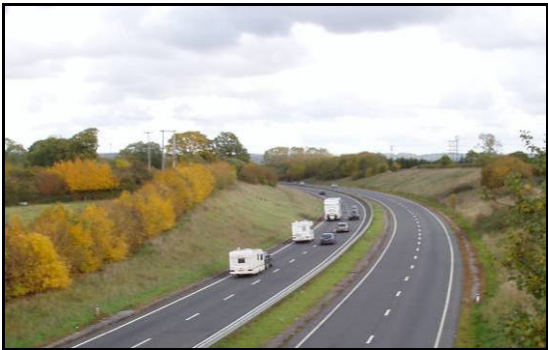
9 The by-pass (A303) looking East
