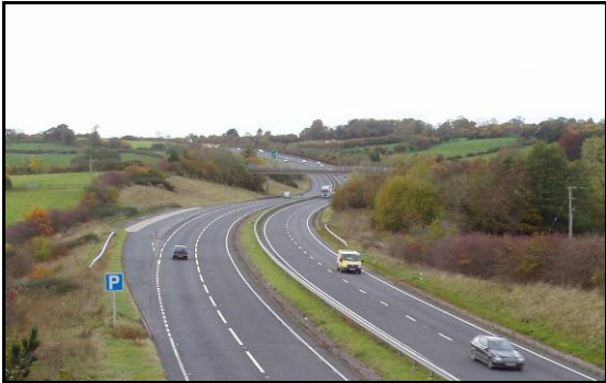
10 The by-pass (A303) looking West
