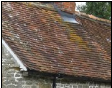
35 Plain tiled roofs at Dovehays Cottage
