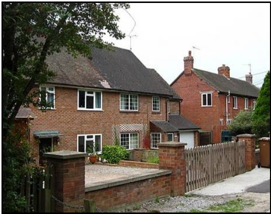
38 Brick elevations at Tan Lane
