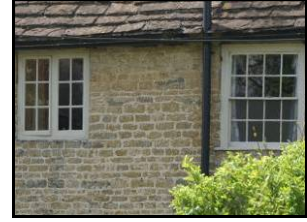
45 Adcroft House windows
