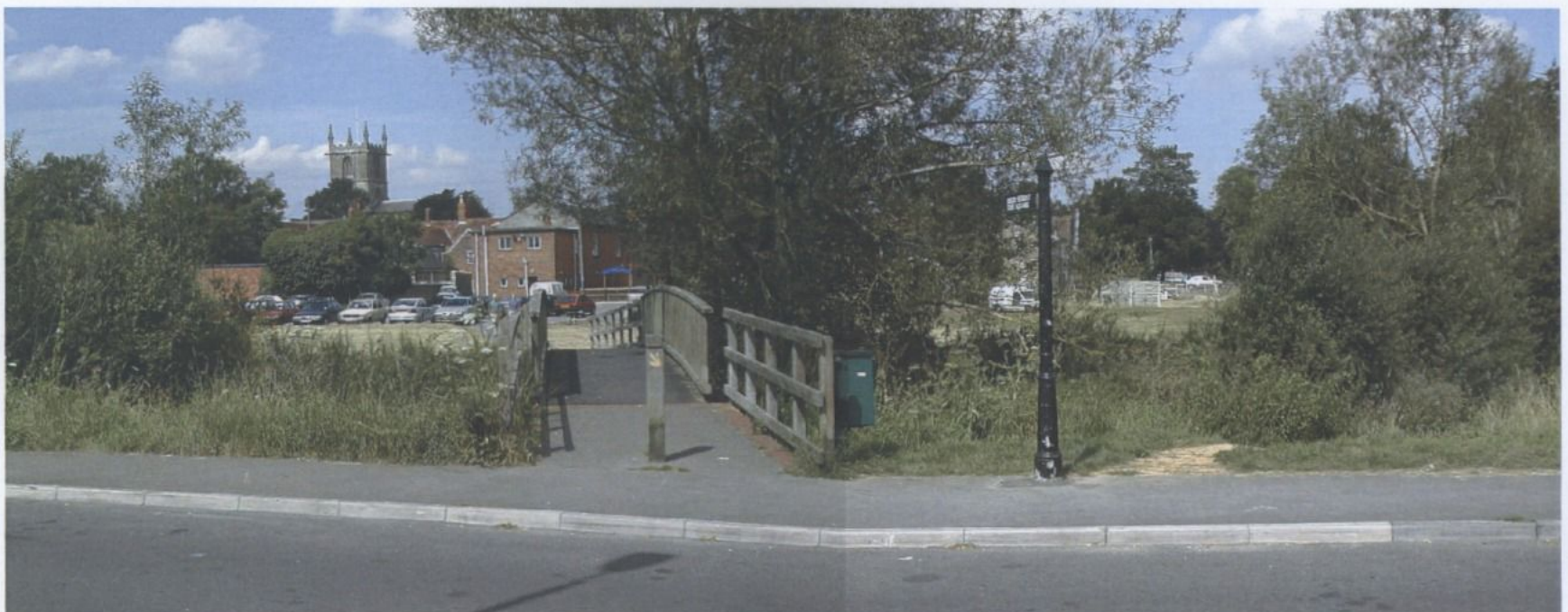
Footbridge from Red Lion to Waitrose
