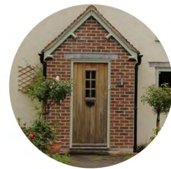
RED BRICK/TIMBER PORCH
