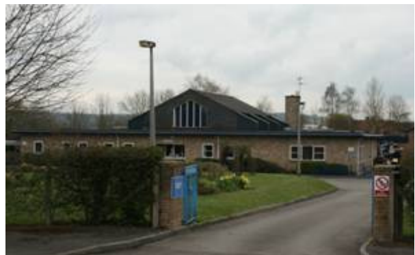
Figure 95: Yewstock School, Honeymead Lane.
