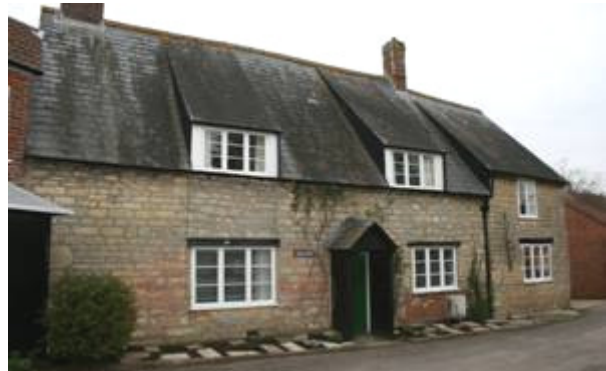
Figure 53: Ham Gate Farmhouse.
