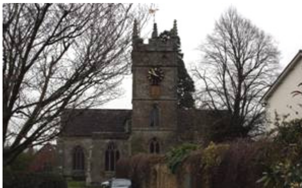
Figure 49: View of the west front of St Mary's Church.
