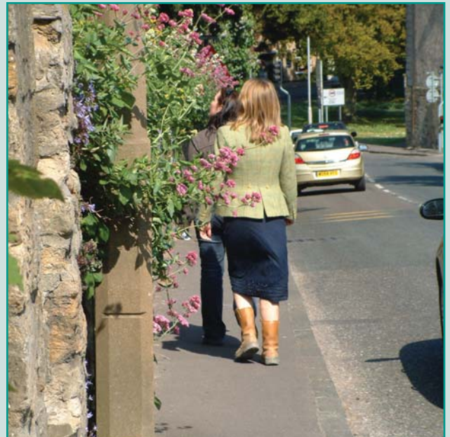
Pavement width confined by listed wall, Sherborne
