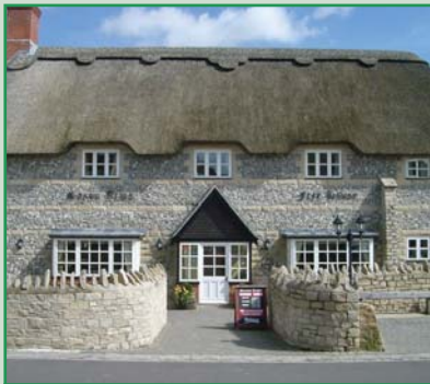
Flint and limestone walls, thatched roof, Stratton
