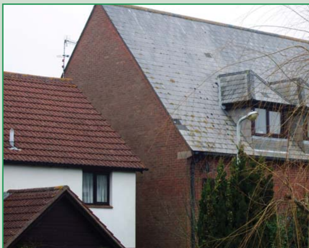
Consider how pitch relates to adjoining buildings
