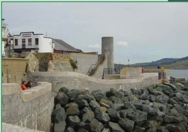
Creative design of storm tanks and sewage pumping station in Lyme provided public open space along the sea front
