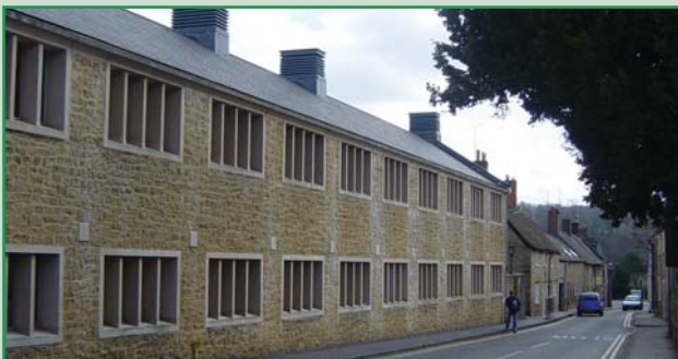
Contemporary chimney vents in new build, Sherborne
