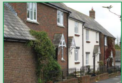
Brick and rendered walls, slate roofs, Chickerell
