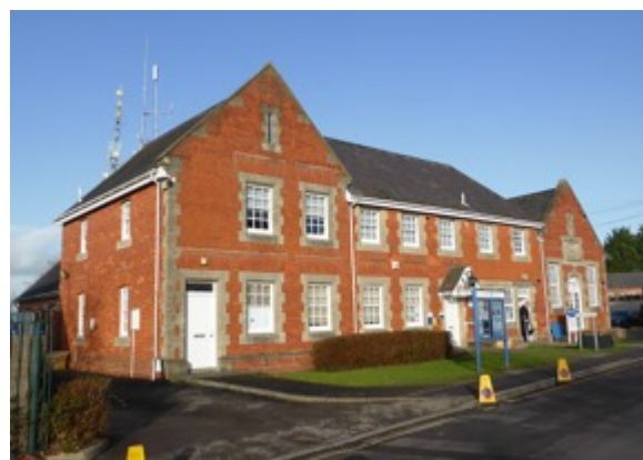
Town Hall and Police Station
