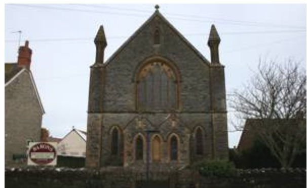
Figure 52: Methodist Chapel, Ring Street.
