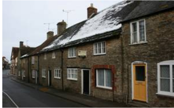
Figure 24: Eighteenth century cottages, Ring Street.
