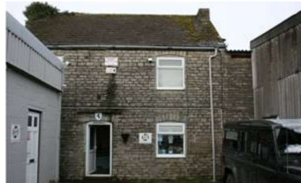
Figure 27: The old Gas Works, Station Road.
