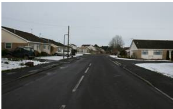
Figure 29: View of Jarvis Way bungalows.
