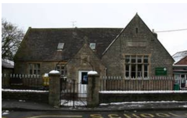
Figure 34: Stalbridge Primary School, Duck Lane.
