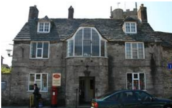
Figure 44: The Town House, The Square.
