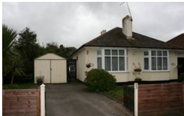
Figure 52: Avon Park Housing Estate
