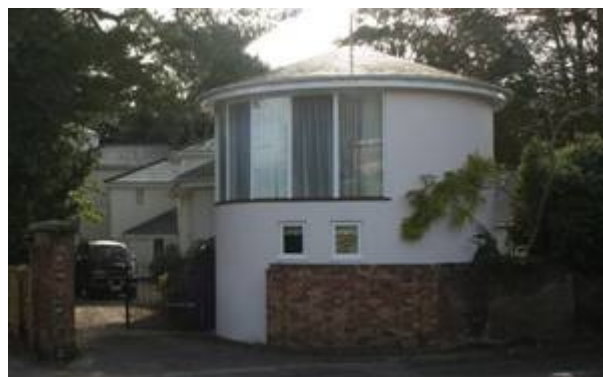
Figure 57: Modern buildings at Mudeford
