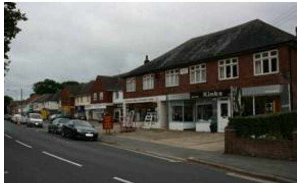
Figure 55: Grove Housing Estate
