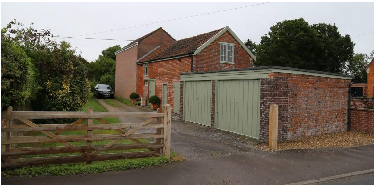
Restored property and outbuilding, Foster's Hill:
