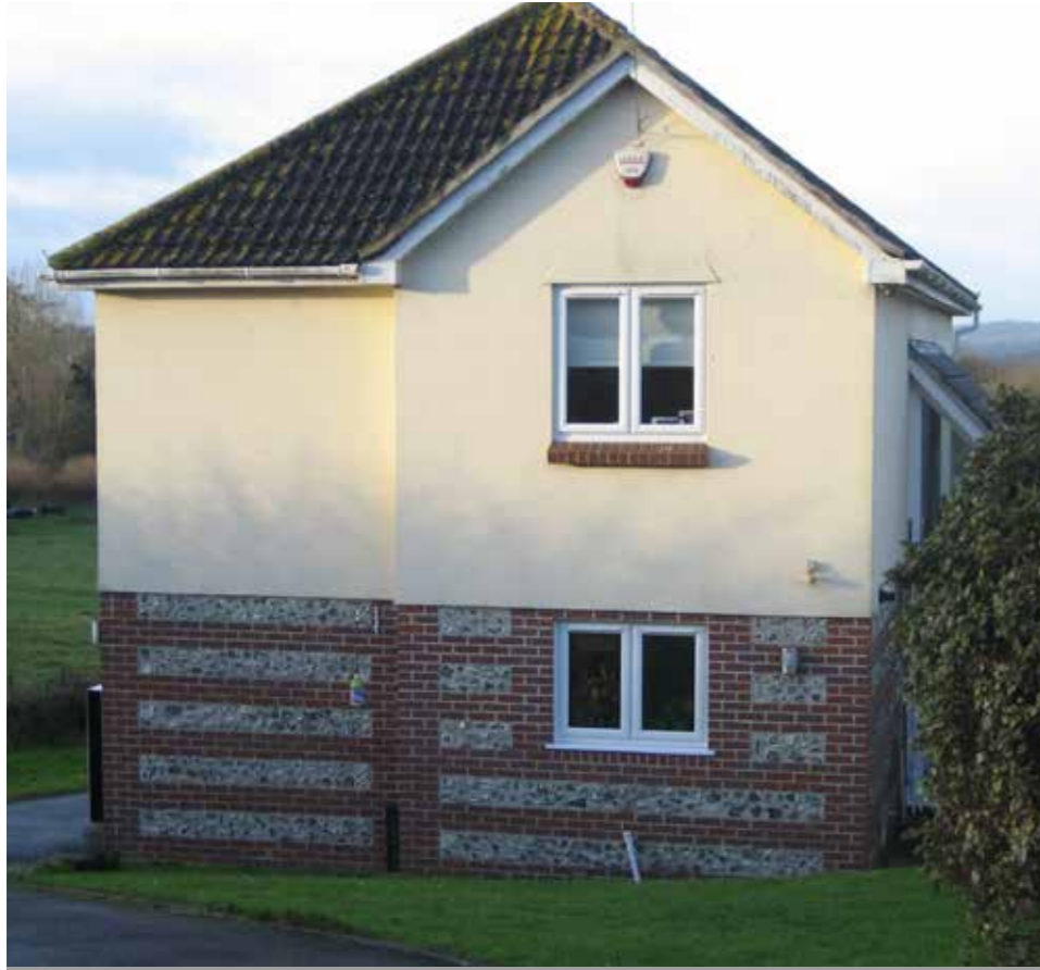
Alteration of facade materials: rendering, stone and brick.
