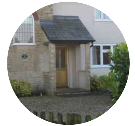
BRICK PILLAR PORCH
