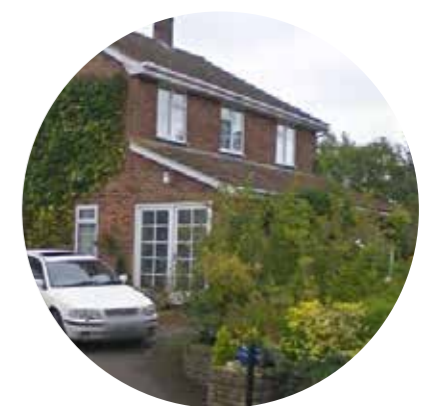
WINDOWS ON ALL FACADES
