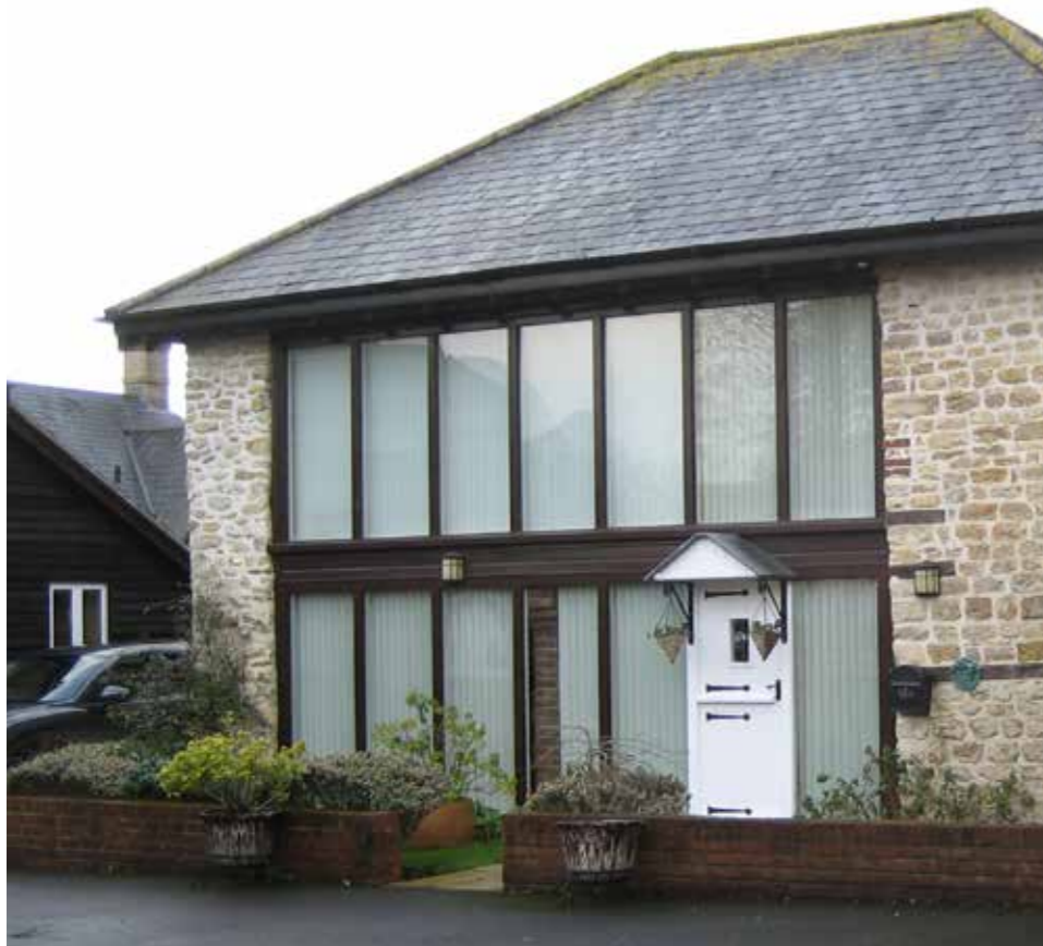
Different typologies of contemporary take on windows. Combination of fixed glass ribbon window with casement of front door.
