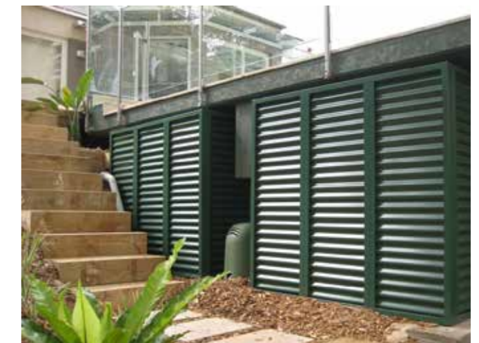
Fig K4 Rainwater tank: integrated design.
