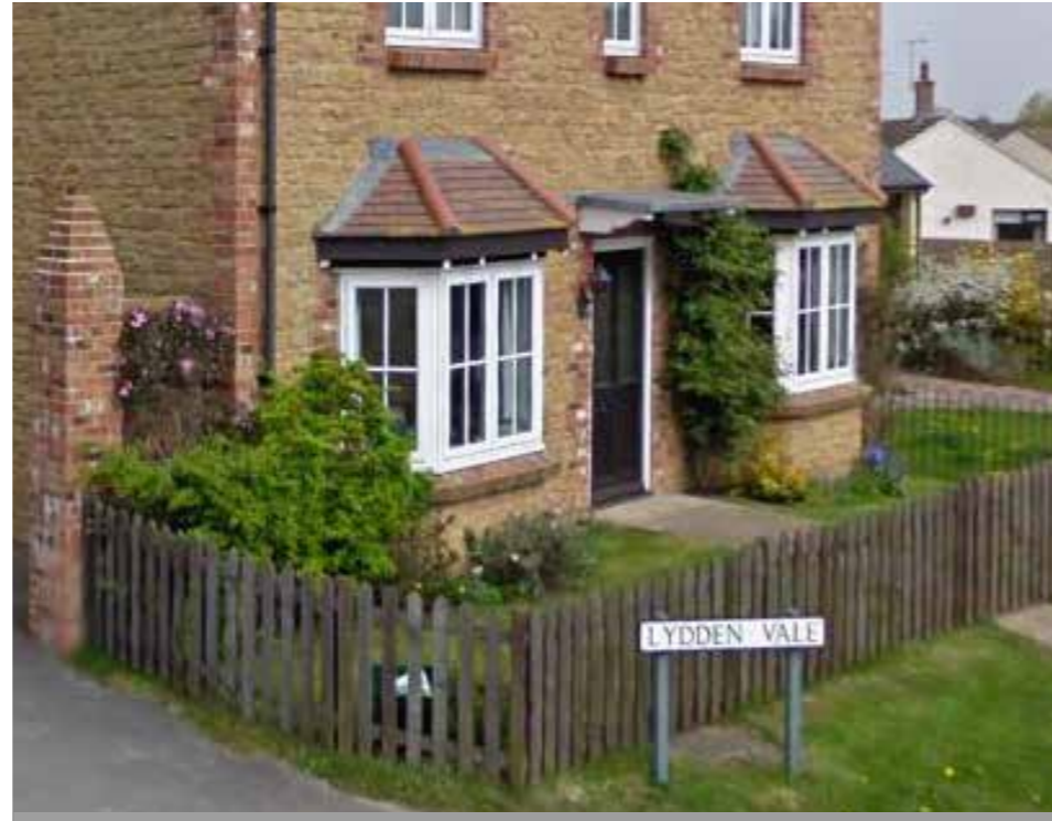
Fig J1 Local examples of typical architectural detailing: bay window.
