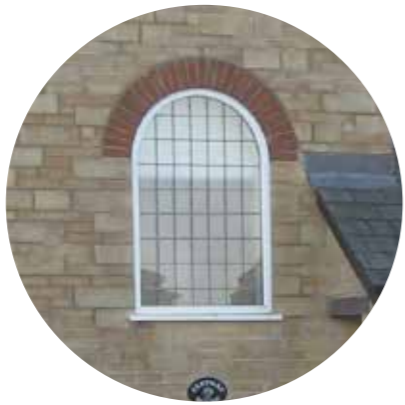
MASONRY DETAILING /ARCHED WINDOW
