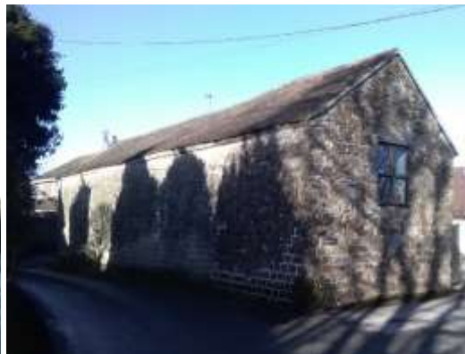
Cross Cider Barn East
