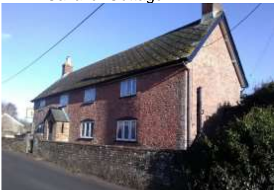
Cavalier Cottage promenade roof tiles and fine brick boundary wall
