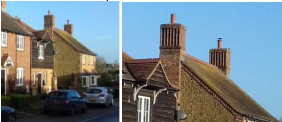
Chimney detail surmounting a stone double fronted house with brick dressings
