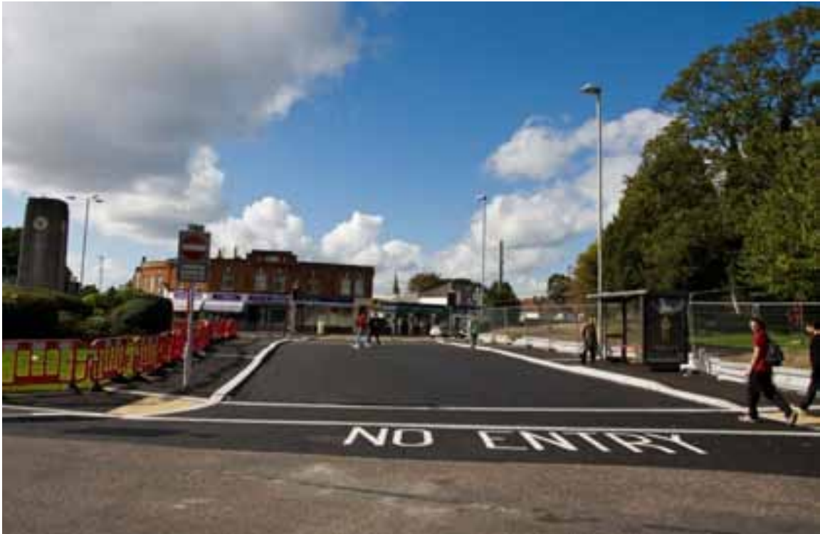
Figure 6.6 – Contra Flow Bus Lane at Poole Civic Centre
