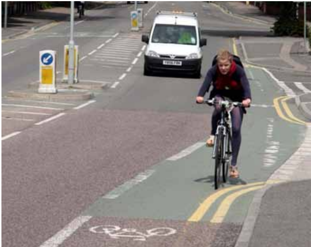
Figure 5.4 – Lansdowne Road Cycle Lane
