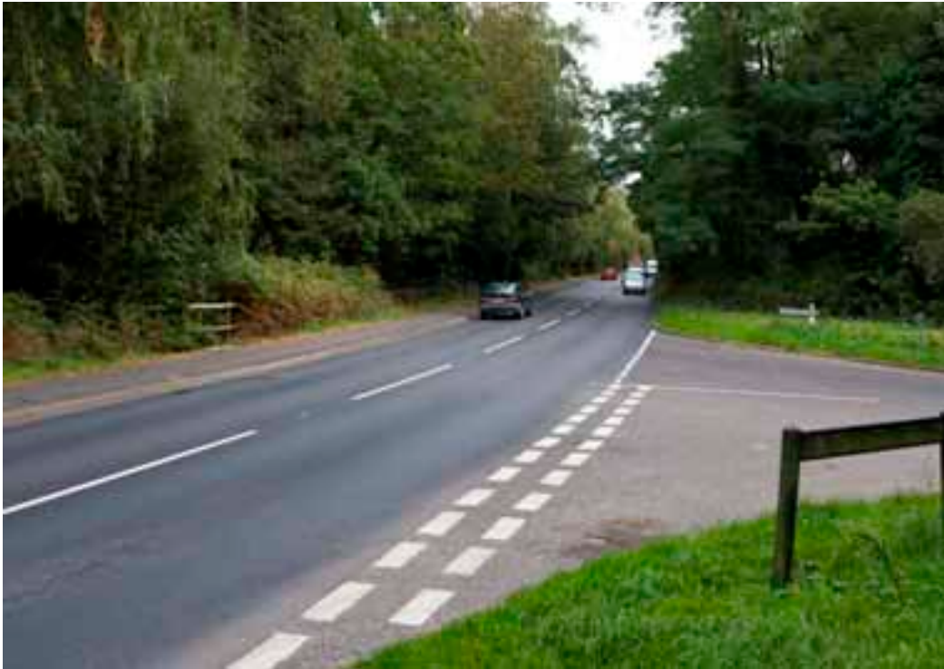
Figure 8.37 – B3073 at junction with Hurn Court Lane looking south
