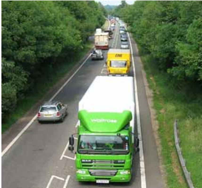
Figure 8.28 – A31 at Merley looking north-east
