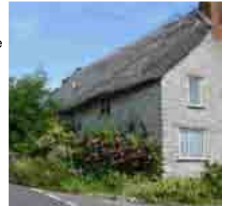
Fig 25. Nos 23 & 25 Front St
