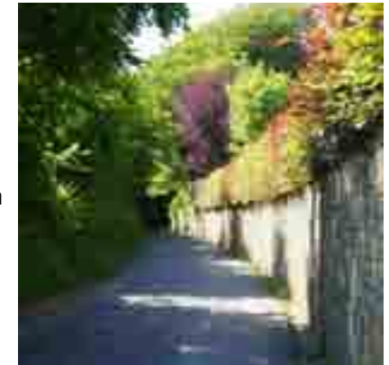
Fig 15. Boundary wall at Langebride House
