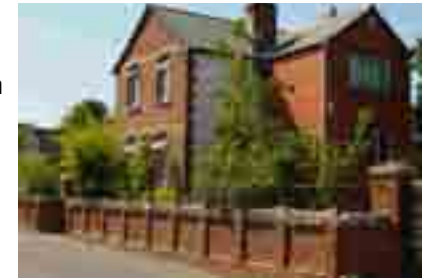
Fig 41. No 61 East St - brick panelled wall
