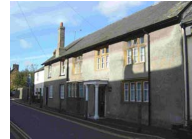
Fig 27. Kingsley House, No.46 Dorchester Rd
