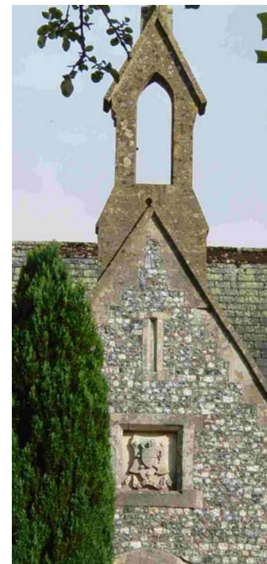
Fig 2. Former school, Frampton
