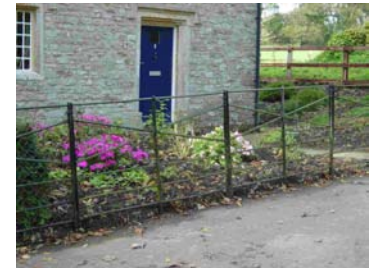
Fig 20. Estate fencing, an example of ironwork
