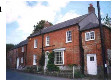
Fig 56. Culvers, Duck St
