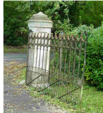
Fig 50. Cast ironwork of Peacock Lodge gates
