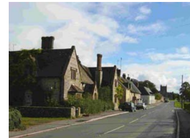
Fig 39. Almost continuous line of buildings on Dorchester Rd (Northover)
