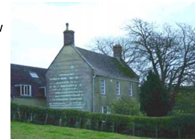
Fig 64. The Old Rectory from public footpath S22/1
