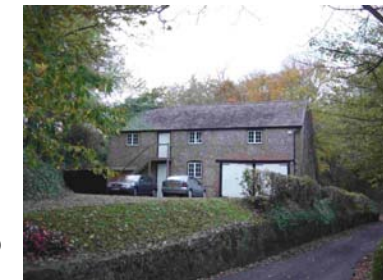
Fig 74. Ancillary building west of Grove House
