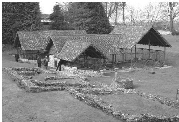
Fig 4 The Roman Town House in Colliton Park was discovered in the late 1930's. The cover building was erected after re-excavation in 1997-8 & designed by John Stark & Crickmay Partnership.
