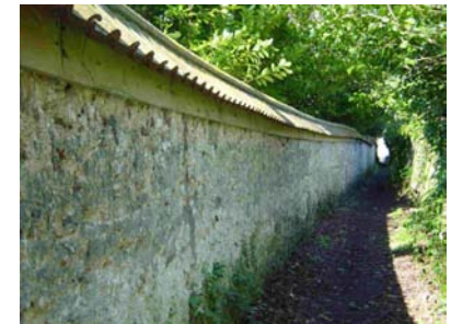
Fig 33. Cob & pantile boundary wall to Charminster House
