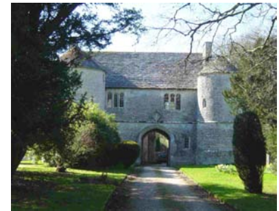
Fig 43. Gatehouse of Wolfeton House
