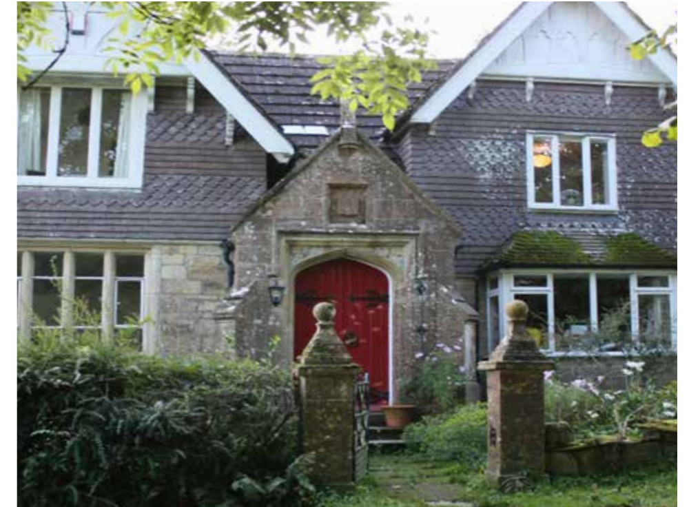
Fig 3.2.22 Local examples of typical architectural detailing.
