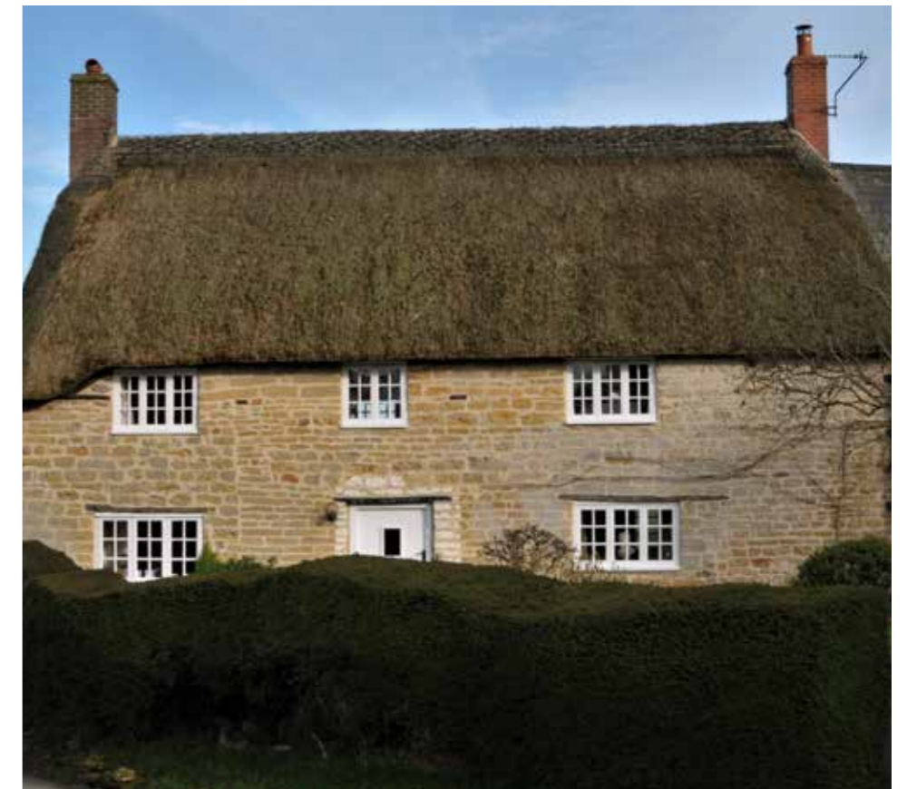
Fig3.2.23 Local examples of typical architectural detailing
