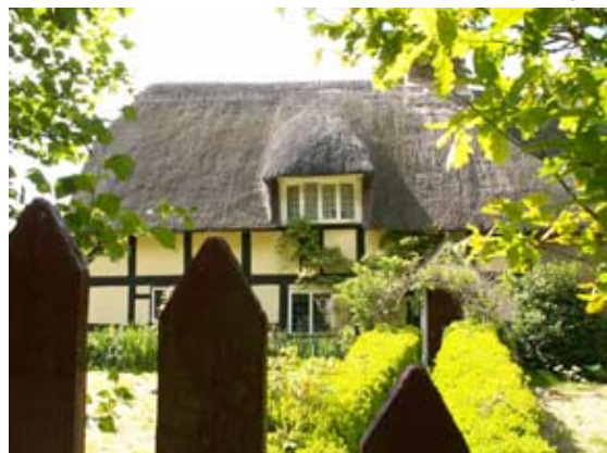
No. 542 Abbott Street, a Grade II Listed Building
