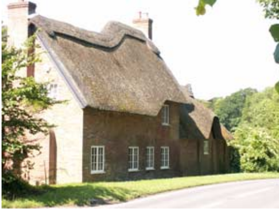
Former estate workshops, a Grade II Listed Building
