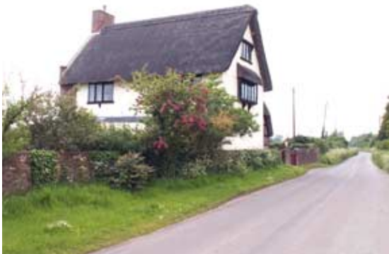
Court House, a Grade II Listed Building
