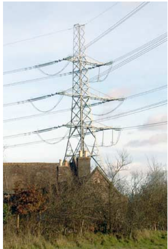
400kv overhead line & pylon at Little Pamphill
