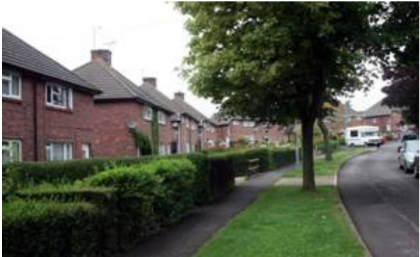
Figure 155: South Avenue, Lenthay Road
