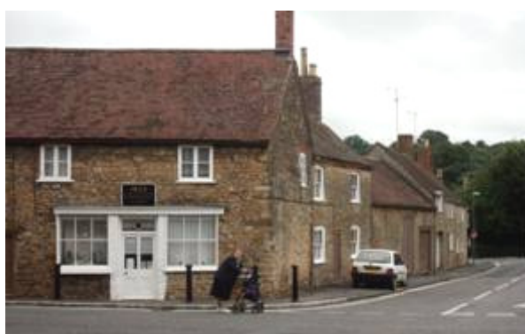
Figure 136: View south along Lower Acreman Street from the junction with Trendle Street
