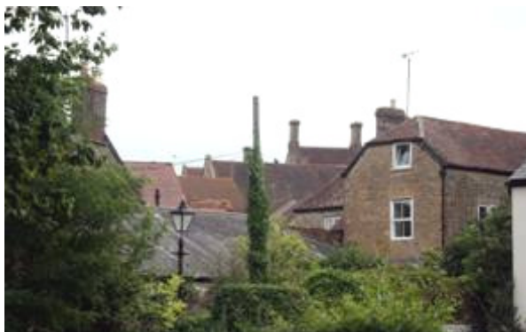
Figure 138: Westbury roof line looking south east
