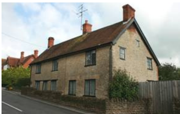
Figure 95: Old Toll House, Wyke Road.
