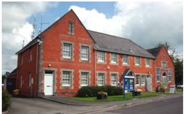
Figure 52: Gillingham Police Station and Town Hall, School Road, Newbury.
