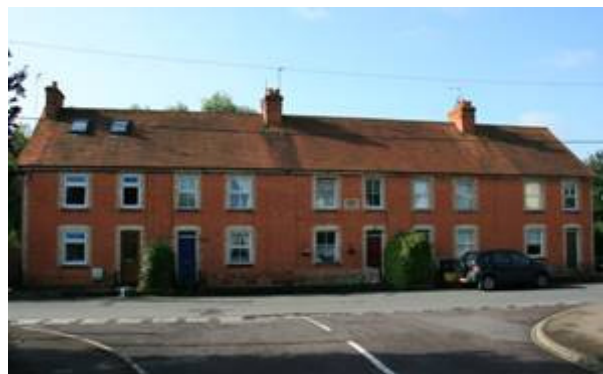
Figure 44: Elm View Terrace, Bay Road, Lodbourne.
