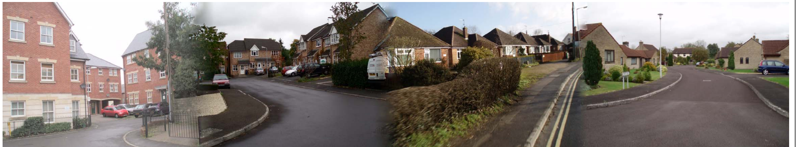
Building Heights – ranging from four storey to single storey bungalows.
