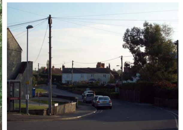
Overhead electricity and telephone lines and poles in Bay Lane
