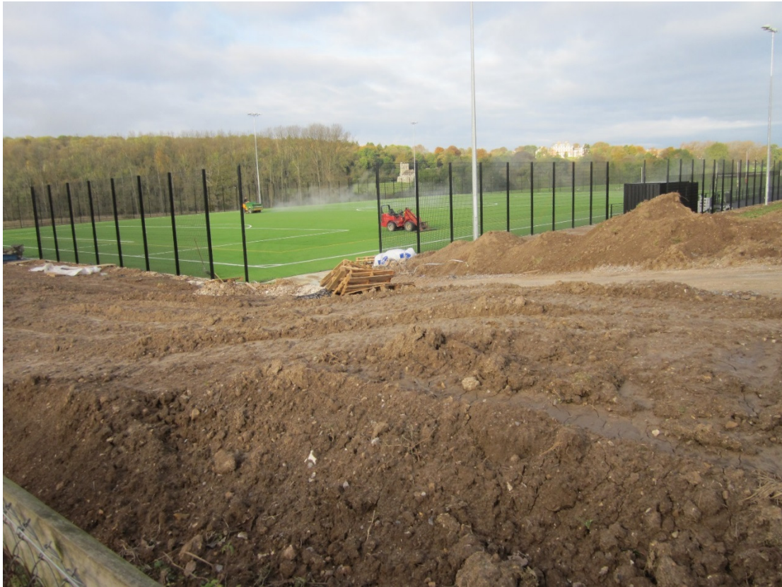
5. View of newly constructed all-weather pitch looking north west to Bryanston Church
