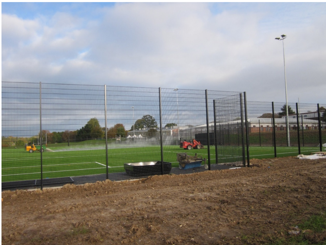
6. View of newly constructed all-weather pitch from within the site
