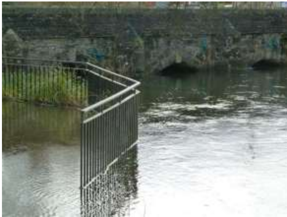
Figure 1 - West Face of Walford Bridge
