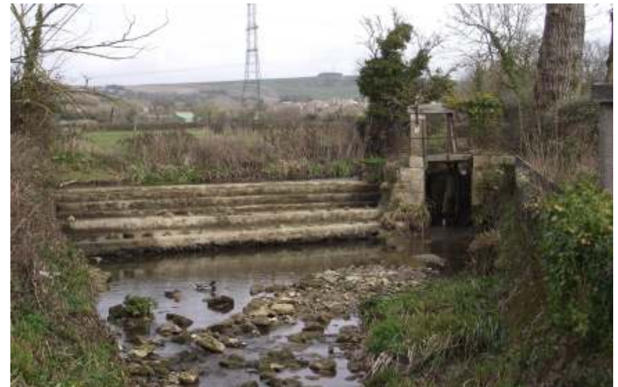
Plate 8 - Weir and sluice to south west of Spa House. Abandoned element of water meadows.
