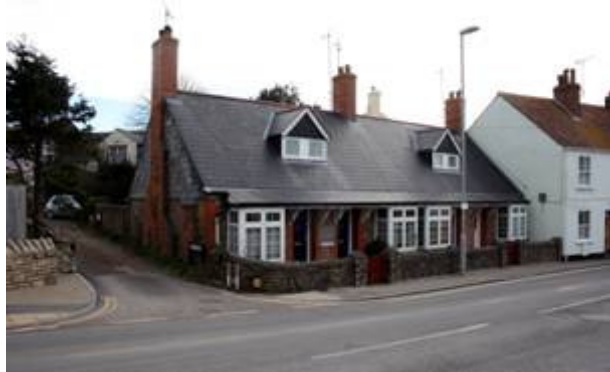
Figure 12: Tubold Almshouses, Church Street.
