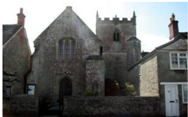
Figure 34: St Edwards Catholic Church, Salisbury Street.
