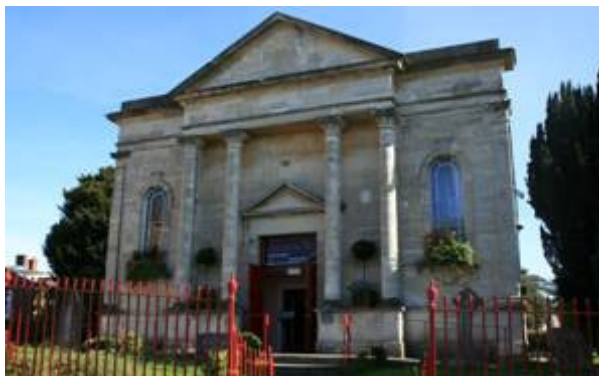
Figure 33: Former Congregational Chapel, Muston's Lane.
