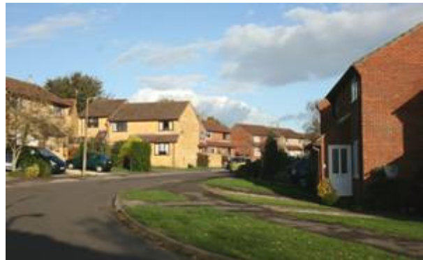
Figure 110: Modern housing estate, St James.
