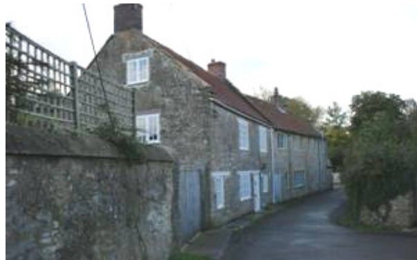
Figure 74: Flax Mill Cottage, 3 Shorts Lane, formerly David Bugler's Bag Manufactory, early 19th century.
