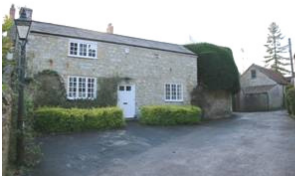
Figure 75: Knowle Cottage, 1 Shorts Lane.
