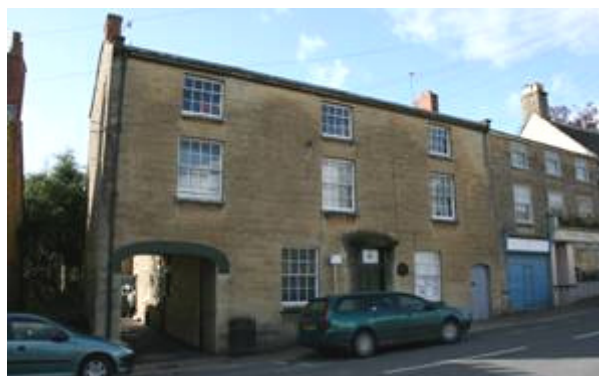
Figure 24: Former 19th century Police Station and Magistrates Court, 6 Prout Hill.
