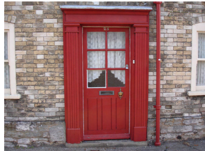
2. A house finished in the livery of 'Rempstone Red'.
