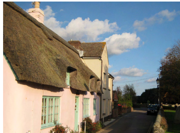
1. Some thatched buildings survived the fire and remain to the present day.
