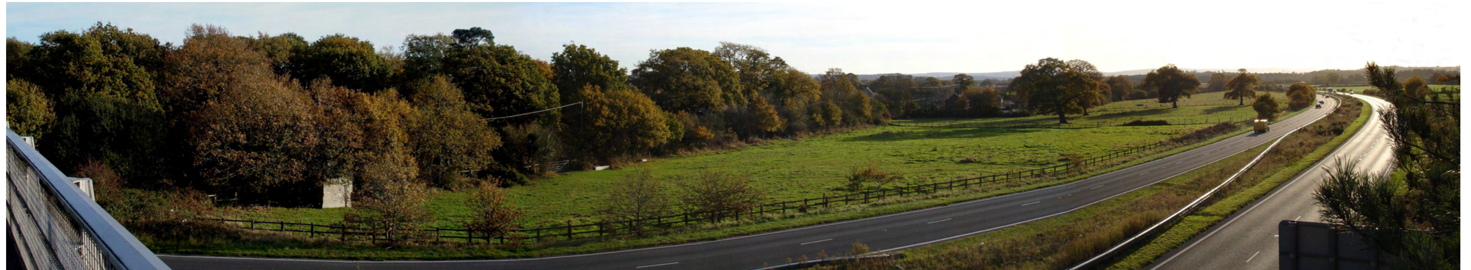
3. The western edge of Upton seen from the B3067 bridge over the A35 dual carriageway. This photograph demonstrates the well-contained edge that visually separates suburban sprawl from adjoining open countryside and the rural village of Lytchett Minster, off view to the right. The established hedgerow/woodland belt contains many mature oak trees and it makes a particularly successful and appropriate edge and screen to what is, in effect, the westernmost edge of the Poole/Bournemouth conurbation.
