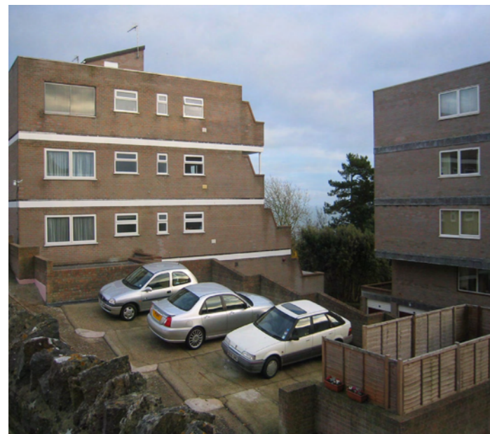
3. A flat development taking advantage of changes in ground level to provide 4 and 5 storey buildings.
