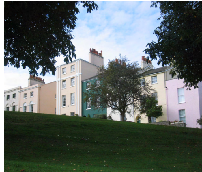
2. Areas of critical townscape largely relate to those parts of the town with high architectural and historic interest.
