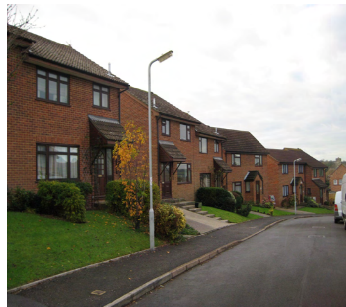
4. Large areas of the town, notably, later large scale housing estates, represent ubiquitous forms of development and are identified as areas of tradable townscape.
