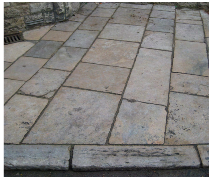
3. Many of the more historic streets have Purbeck stone paving and kerb detailing. This is particularly prevalent along the High Street, but even some late 20th century estate roads have Purbeck stone kerbs.
