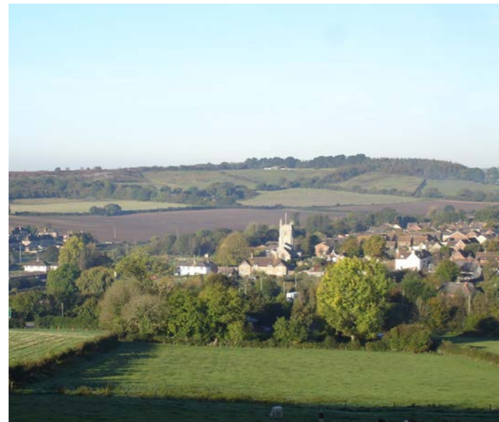
1. The church is the tallest and most prominent built feature of Bere Regis despite being situated on low ground.
