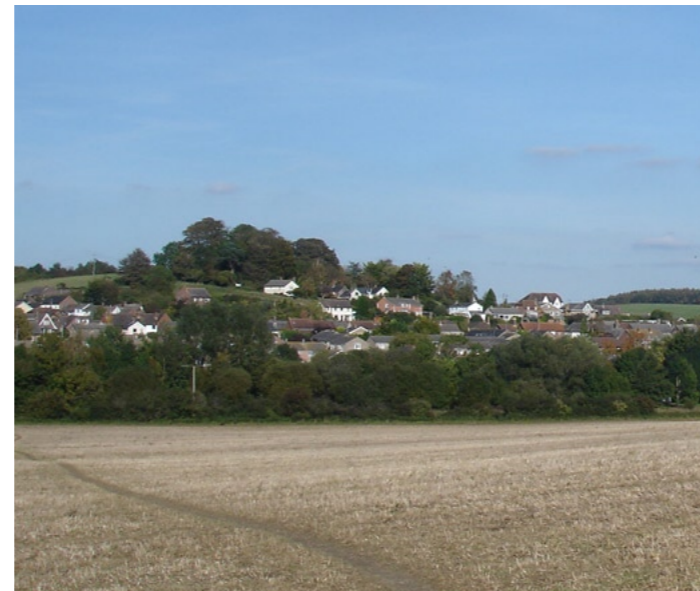
2. A pleasing composition of roofs on the side of Barrow Hill.
