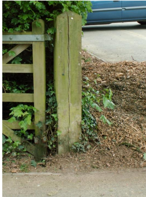
Figure 40: A long range pyro at a Borough of Poole site
