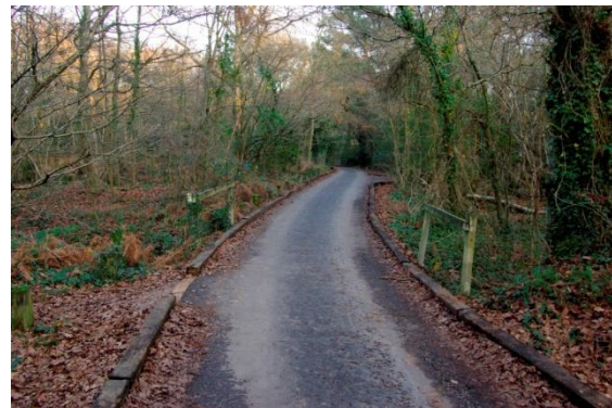
Figure 14: Access drive at Delph Woods after project completion
