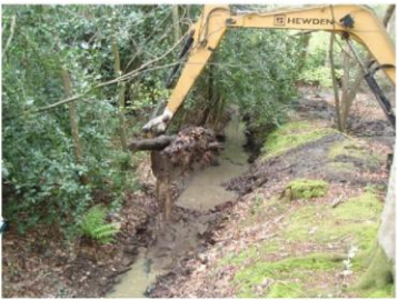
Winter 2008/09 Ditches are cleared and re-profiled
