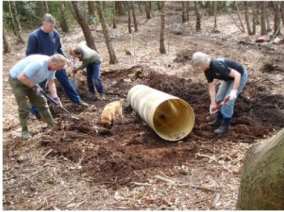
March 2009 An old fibre glass play tunnel is salvaged and installed on site. A trench was dug and then the tunnel put in its place and backfilled. Tommy liked walking over rather than through it!!
