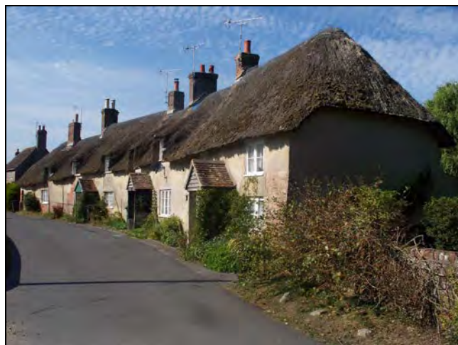
FIG. 13: Thatched roofs of Nos. 2-5 The Street.
