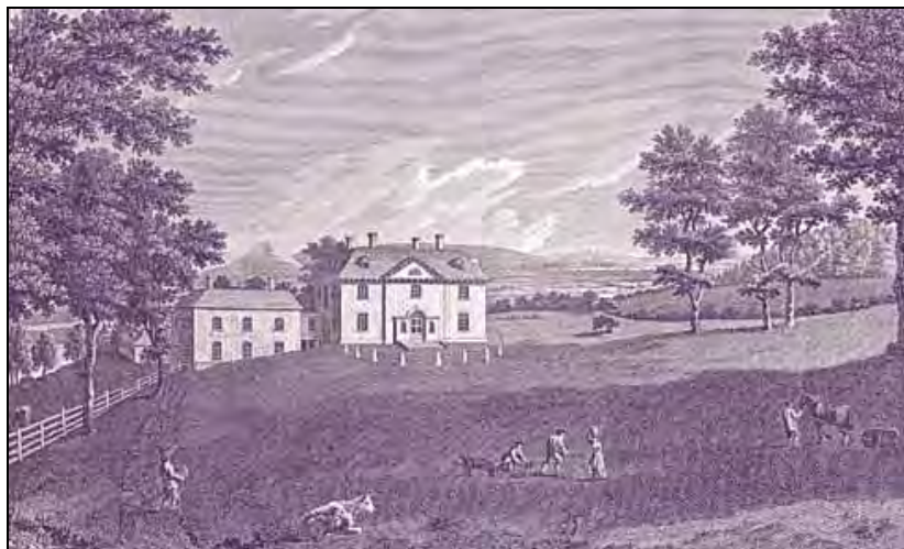
FIG. 1: Moreton House c.1774. From the first edition of Hutchins. Compare with the view in FIG. 3, which shows little change. Whilst some artistic license must be allowed for, details such as the subdivision of the parkland with post and rail fencing and the generally open (heathland?) backdrop are of some interest in understanding past landscape character and management.
