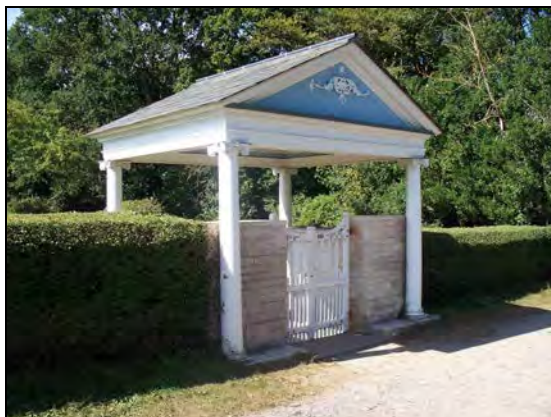
FIG. 4: Classically styled gate to the new cemetery. Originally constructed c.1800 as entrance to the kitchen garden, and moved here c.1950. The modern brick walls either side incorporate panels taken from the obelisk on Fir Hill to the south of the conservation area.
