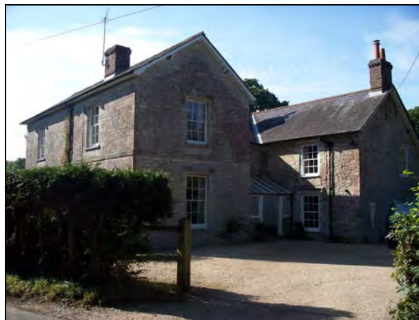
FIG. 15: Manor Farm. The original house is the range to the right, and probably dates to the early nineteenth century. The range to the left and centre is a large extension probably added later that century. The quality of construction and retention of many original windows is notable. Reflecting the different dates of the two parts of the property, the windows on the older range have exposed sash boxes, whilst those on the later range are recessed.
